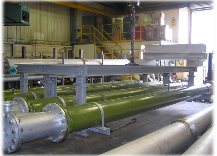
Pipework and support structure fabrication and assembly
