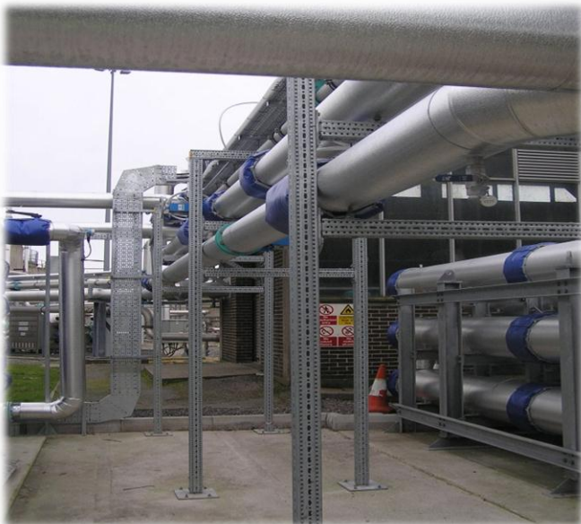
Watermark Fabricated and Installed pipe-work on-site
