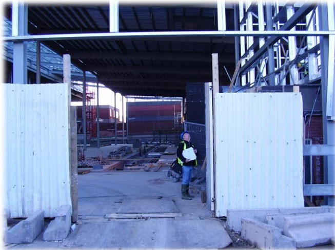
Work on Steel -structure
