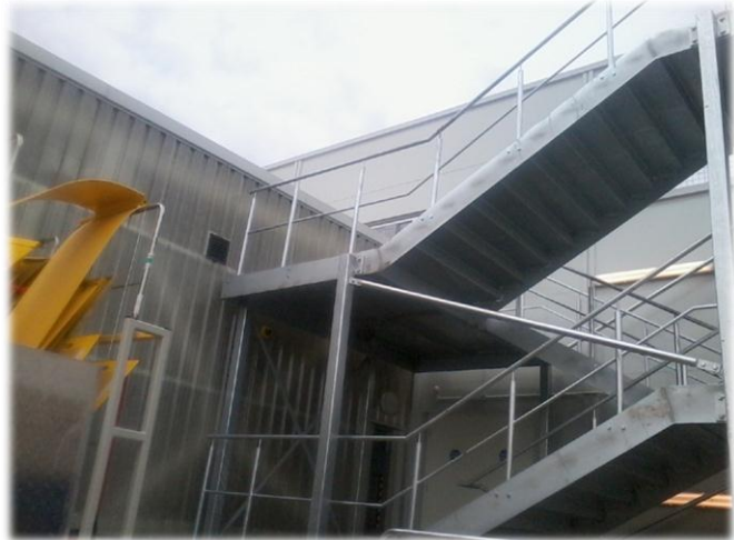
Steel work to staircase
